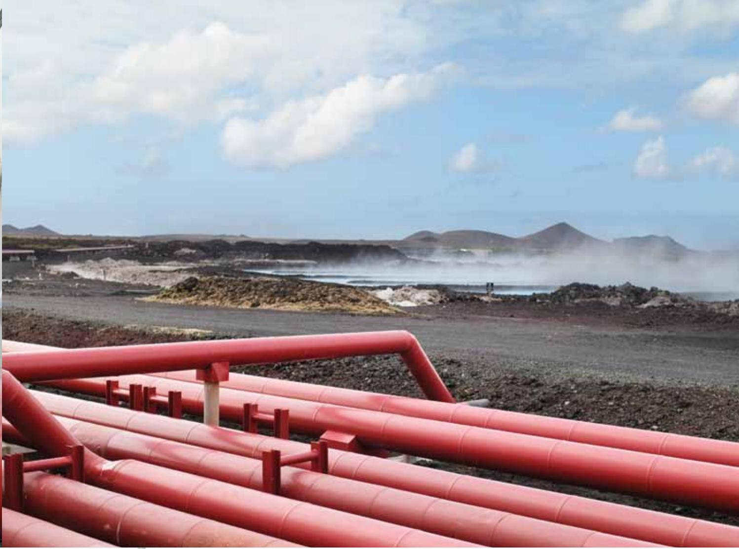
The geothermal plant in Svartsengi started production in 1976 and was the first facility in Iceland to combine electricity production with utilization of the resulting hot water for domestic heating. The plant, situated in the south-west of the country on the Reykjanes peninsula, was built in five stages.
